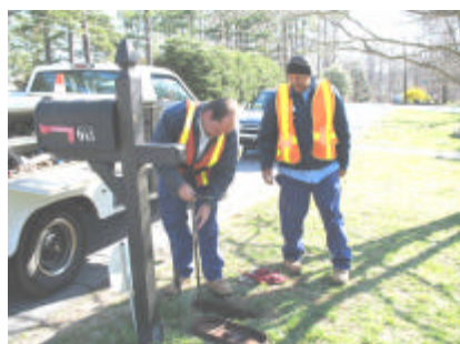
Maintaining water meters
